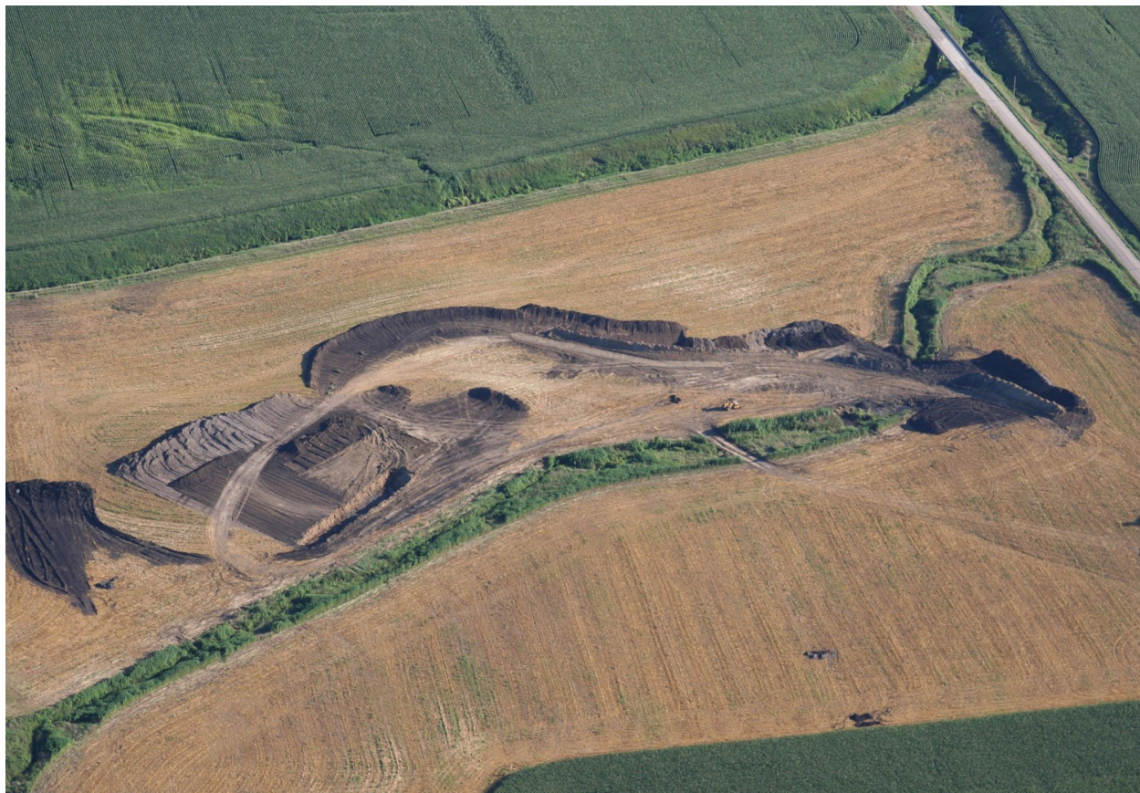
CREP site construction in Wright County, Iowa.
